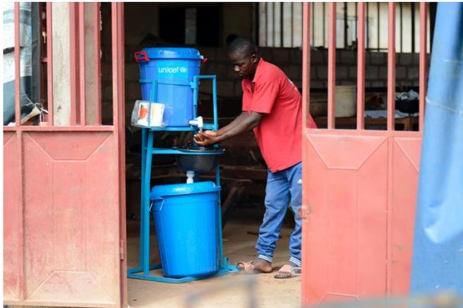
A pedal-operated handwashing facility manufactured with UNICEF support. ©UNICEF/UN258001/BUTA
